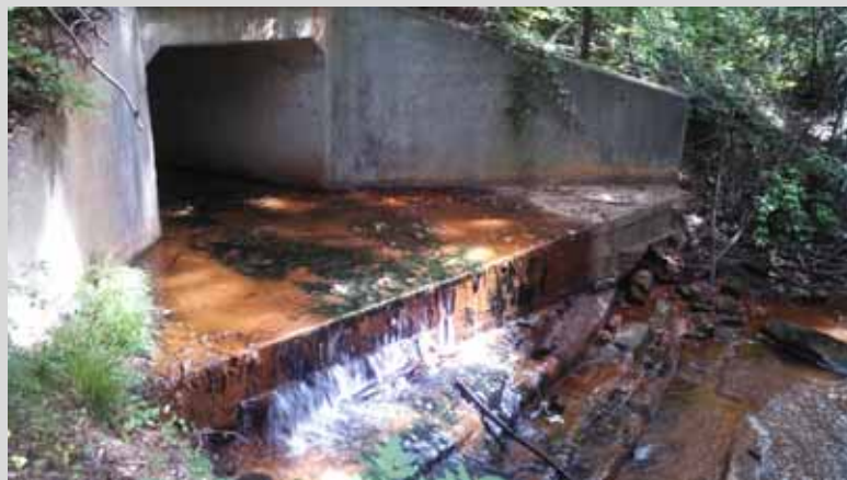
Photo 1. Unnamed Perennial Tributary to Anneewakee Creek between SR 5 and Bright Star Road.
