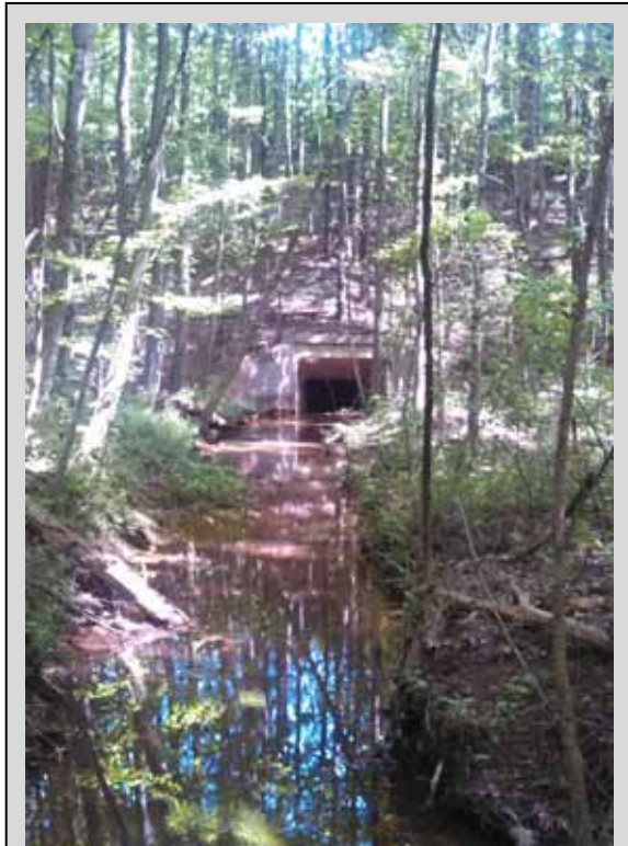
Photo 2. Unnamed Perennial Tributary to Anneewakee Creek under I-20 in Study Area
