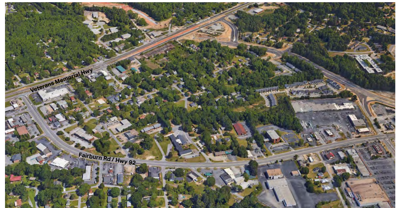
Existing Conditions Aerial of Project Limits
